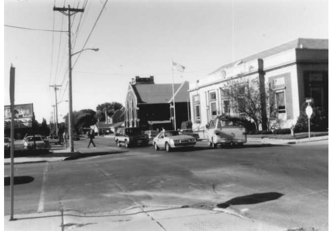
10. Front elevation, looking southwest.
