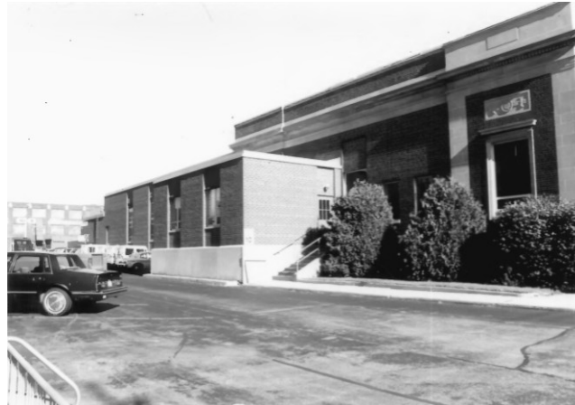
6. Side elevation, looking east.
