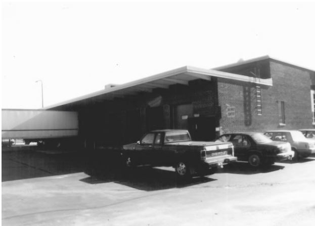
5. Rear elevation, looking northeast.
