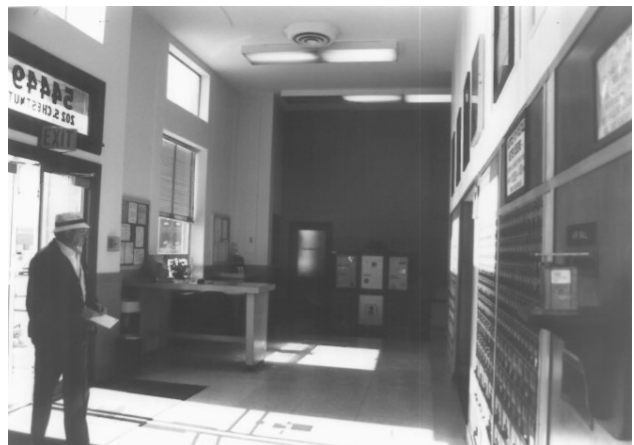
2. Interior view, lobby.
