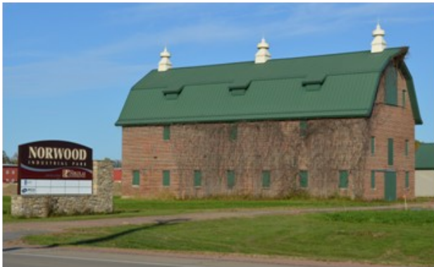
This is the last remaining building of the Wood County Asylum Hospital and Farm complex, also known as Norwood. It is now a part of the Norwood Industrial Park. Photo taken by Vickie Schnitzler, October 2, 2019
