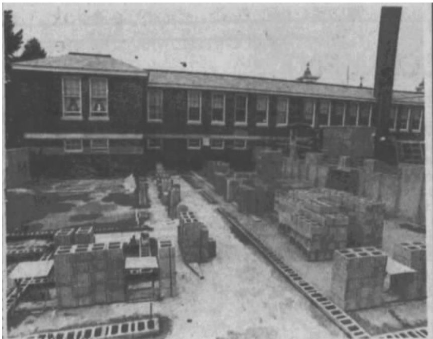
Construction under way
