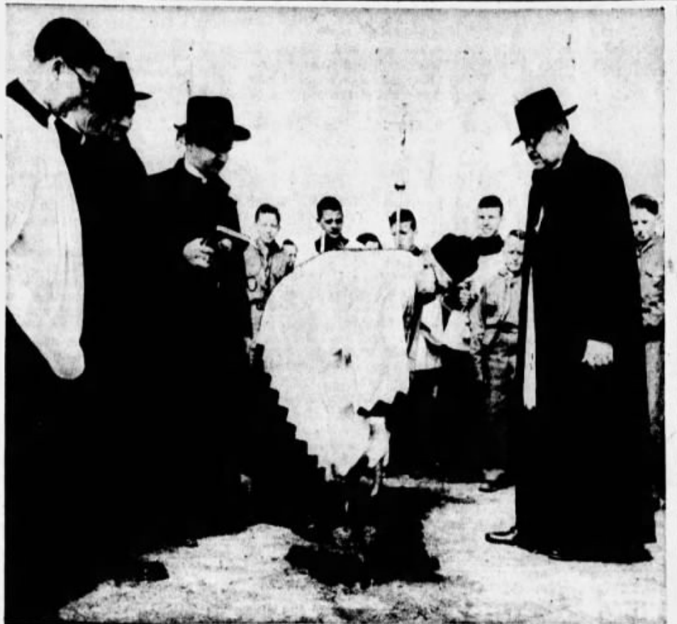
BREAK GROUND FOR CONVENT —Work on the $162,438 convent for Columbus High School and Our Lady of Peace Grade School and Church began officially at 9:30 o'clock this morning when the Rev. Edwin L. Knauf, pastor of Sacred Heart Catholic Church, turned the first shovelful of dirt. Watching the proceedings are, from left to right, the Rev. Richard Rossiter, the Rev. Constant Chilicki, the Rev. James Lane, the Rev. Bernard Schreiber, and the Rev. Walter Dillenburg. The new convent is being constructed on a plot of land between the church and the north end of the high school. (News-Herald Photo)
