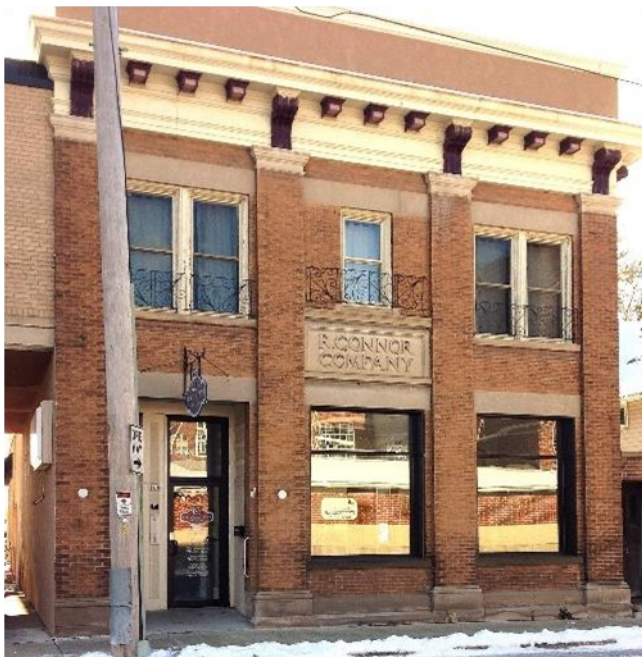
Front view of building.
