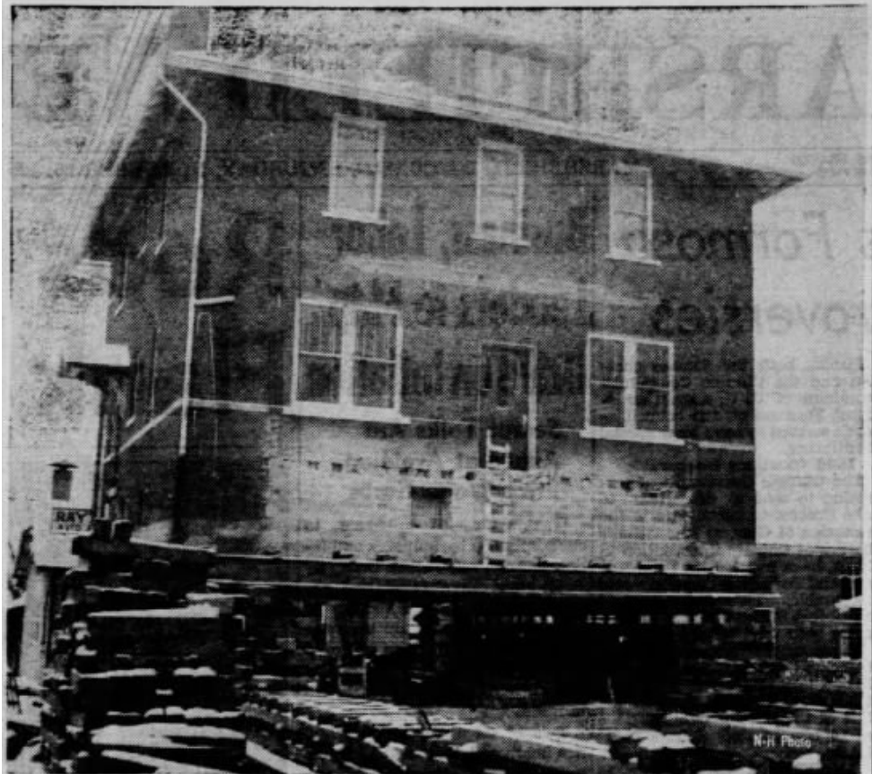
CLUBHOUSE MOVED —The former American Legion clubhouse was moved 44 feet from its old location Wednesday to make room for the Connor Lumber and Land Company building which will be moved in a similar manner. The structure had been raised eight feet before the rollers were put on the steel "saddles" which were supported by timber cribs and pulled into its new position by a winch powered by a truck. After the Connor building is moved back a larger business building will be erected by the firm, facing Central avenue.
