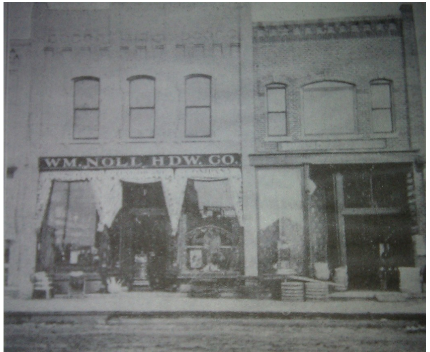
Double store of Wm. Noll Hardware Co. with addition to the south (on right) being built sometime between 1887 and 1891. (photo from Marshfield Illustrated, by C.W. Charles, 1905)
